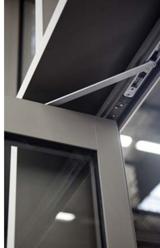
Door spring flush mounted in the upper transom.
