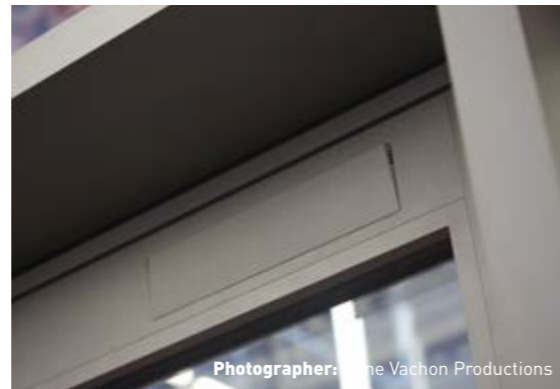
Access hatch for maintenance.
