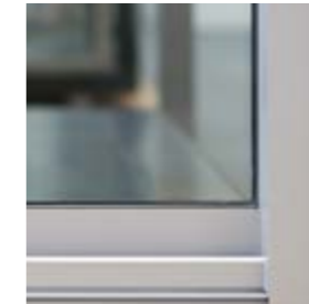
Exterior detail of frame: frame-lower transom
